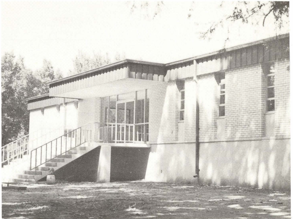
All work of the Kansas Forestry, Fish and Game Commission is administered from the headquarters office building which was constructed in 1965.
